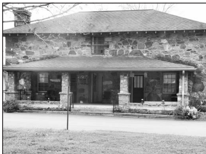
The Old Rock Jail – a historical gem for Towns County – has been restored as closely as possible to its original condition.
